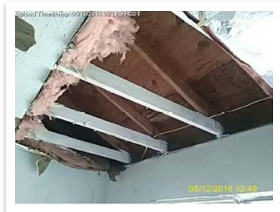
Treatment of studs with stain blocking primer.
