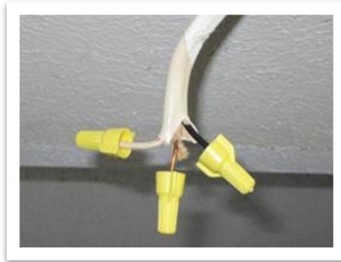
Example of Capping Wires
