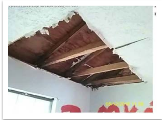
Removal of drywall and insulation.
