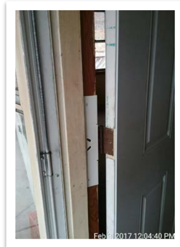
Photo showing door hinge protection product installed.
